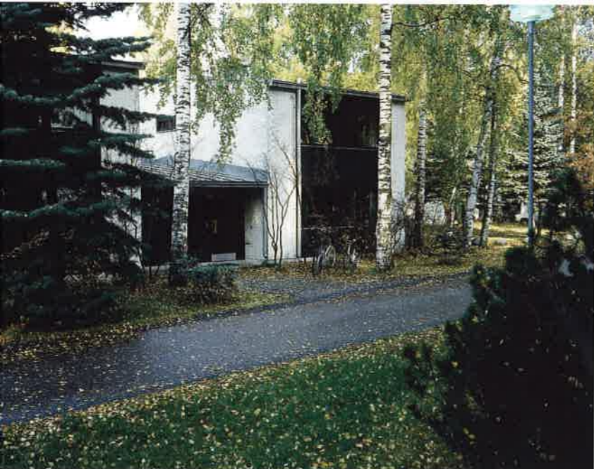
Kaija and Heikki Siren: The Kehräjä row houses (1960). The streetside in October 1984. Photo Riitta Nikula
